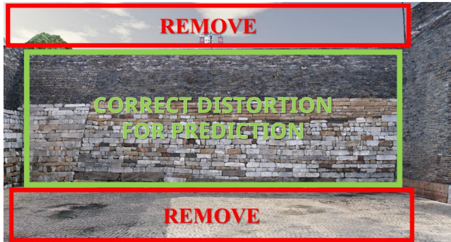
Figure 5: Regions to be removed and to be corrected distortion in the stitched picture.
