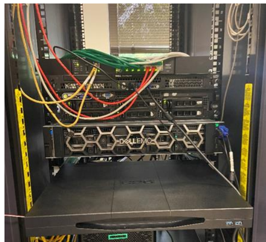
Fig. 4. The 5G Research Testbed. The server labeled “Dell EMC” is the server that will be used for this project.
