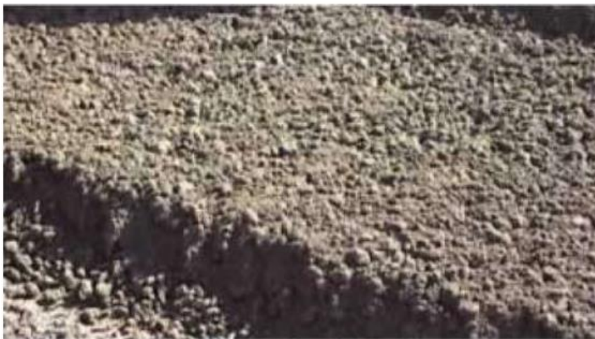
Lime flocculating clay
