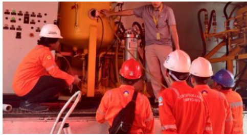
Fig. 6. Reclamation process using PLN machine
