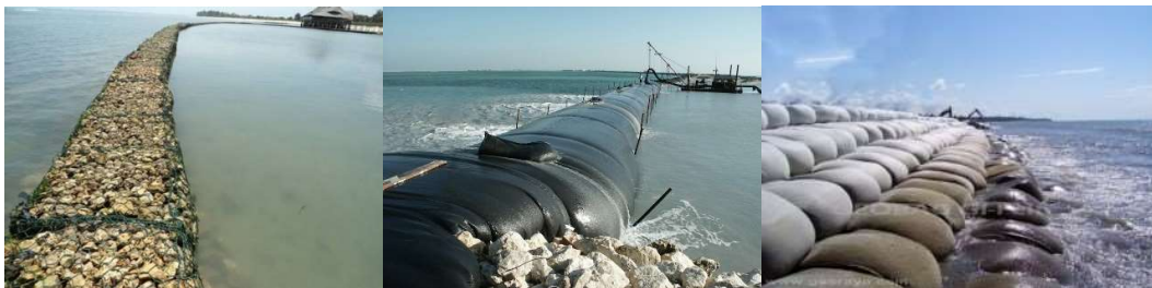
Figure 4. Gabion, Geotube and Geobag type breakwater
